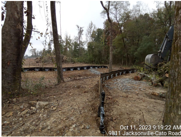
Silt fence and rock check dams at creek/bridge city limit
