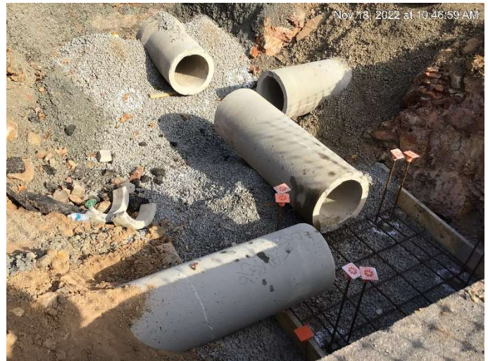
Stormwater Piping @ Fred Raines area Inlet & Junction Boxes
